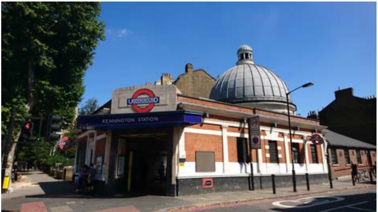
Above: Kennington Underground Station
