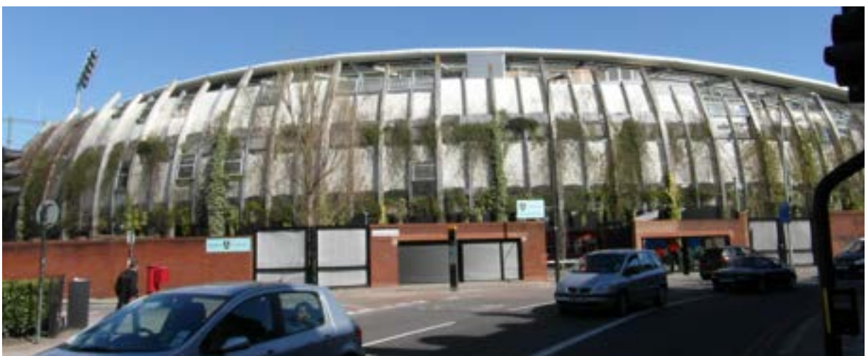
Above: The Harleyford Road end of the Oval
